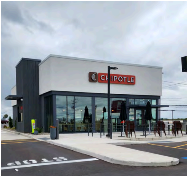
Chipotle restaurant, completed and open
